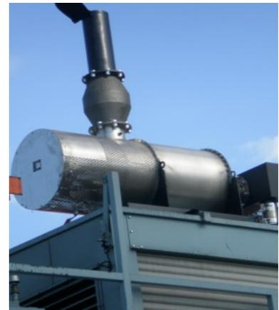
The operation of the RYPOS ActiveDPF/C3+™ is controlled by an advanced electronic control unit, not found in the CARB verified level 2+ system. The DPF uses controlled electric heating for reliable regeneration of the filter cartridges. A diesel oxidation catalyst is added to help remove soluble organic fraction while reducing carbon monoxide and hydrocarbon emissions.
