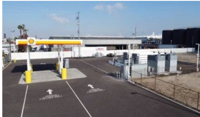
Figure 13: Hydrogen Fueling Station (Wilmington, CA)
