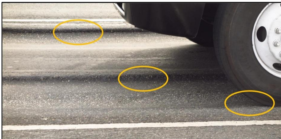
Figure 33 Lane grooves on Alameda Street at intersection
