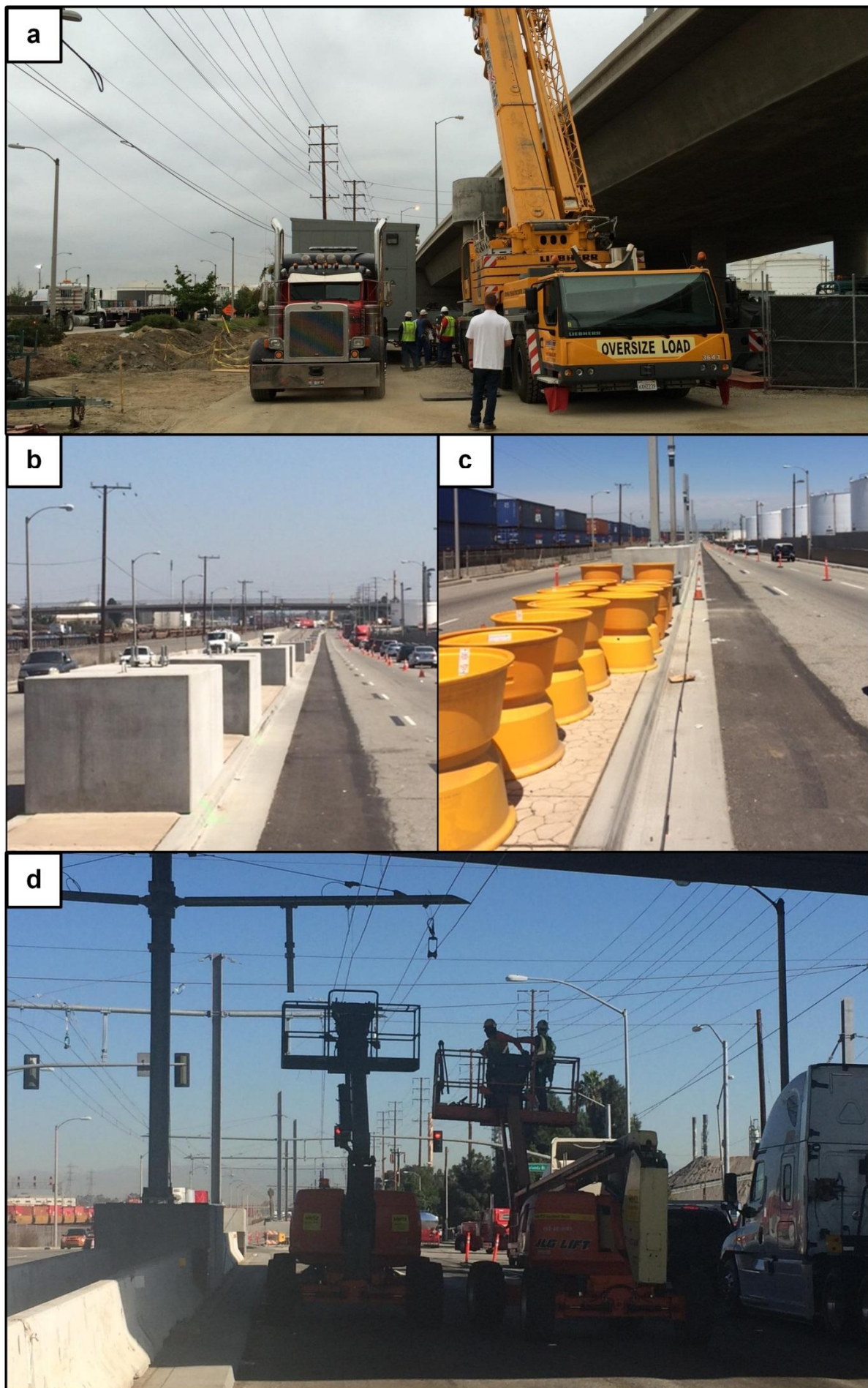
Figure 18 Construction phase – setting of foundations and poles
