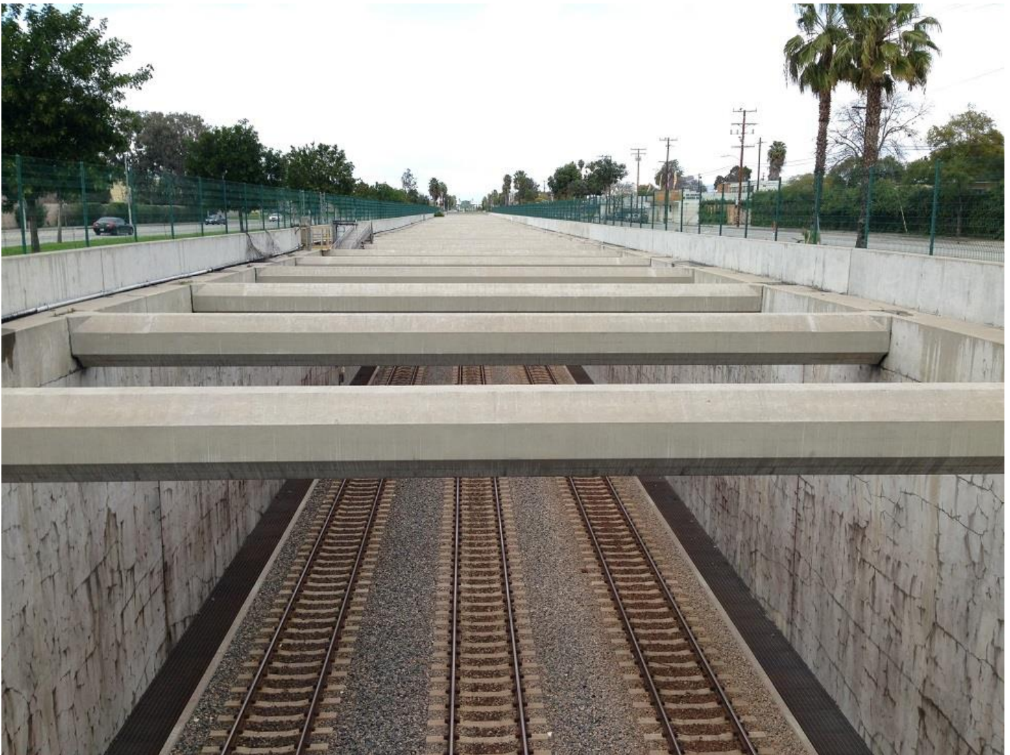
Fig. 3. A section of the Alameda Corridor's mid-corridor trench in the city of Compton. Photo by Brian Yanity
