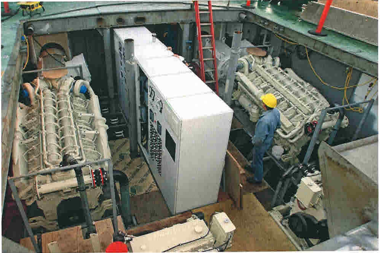
Photo 2: Engine room under construction
