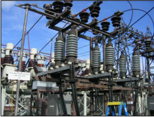
Upgrade 4.8 kV Feeder
