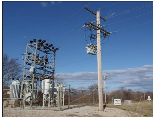
Upgrade 34.5 kV Lines
